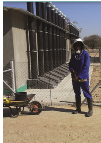
Learners are using Enviro Loo at numerous schools in North-Central Namibia.
